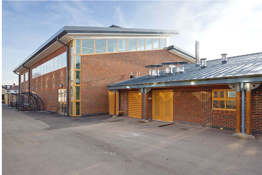
New Hall & Existing Plantroom
